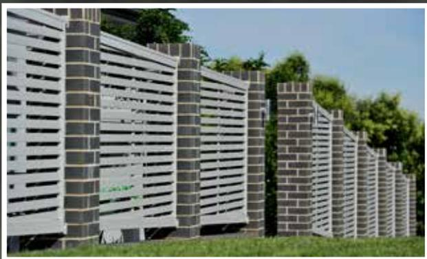
Built from 38x25 RHS frames, 50x10 RHS slats. Choose from a 20mm spacing or a 50mm spacing between slats as a standard range. Custom size spacing is also available. Over 100 powder coat colours to choose from.
